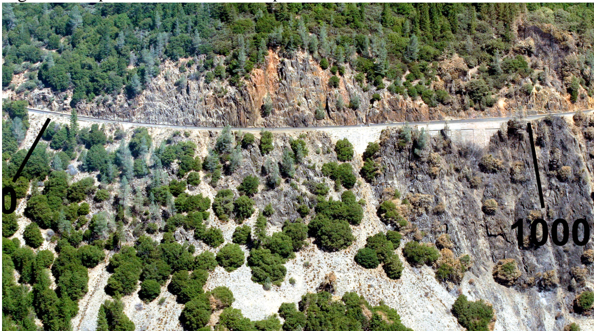
Figure 52 Cape Horn in 2004. Most of the additional cutting and some retaining wall improvements occurred in 1929. After 16 years of abandonment (1913-1929) this roadbed was improved allowing the eastbound, uphill traffic to be removed from Tunnels 33 and 34, and returned to this original 1866 location.
